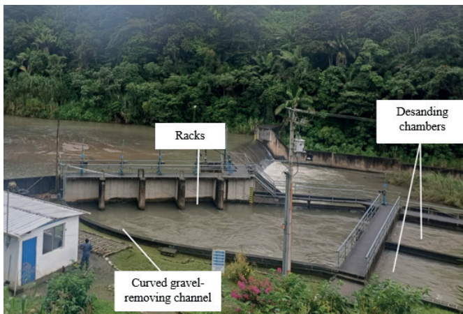
Fig. 3. Analyzed hydraulic structures prototype.
