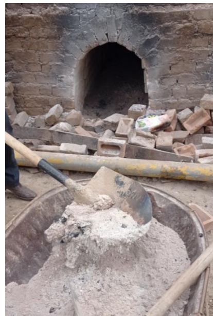
Figure 1. Wood ash extracted from the lower grill area of the brick kiln
